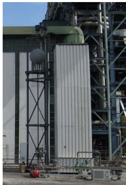
700 kWh (13000 kg) sodium nitrate PCM storage for 300 °C applications (source DLR)
