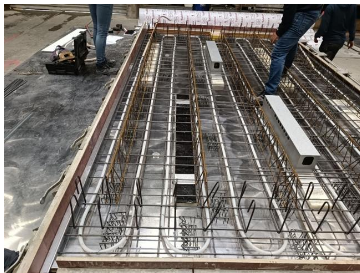
Figure 21: Installation of high-quality building services components in the precast plant, Source: Innogration GmbH
