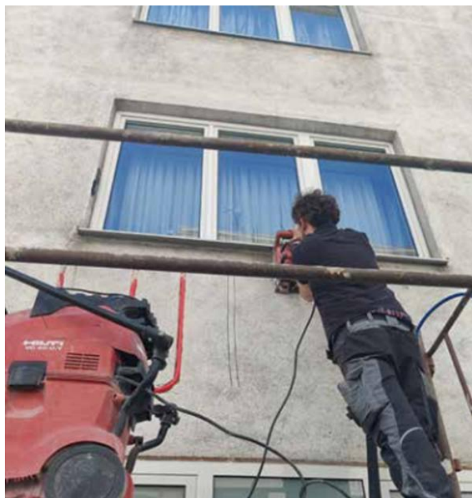
Figure 28: Installation of the heating pipes in the exterior wall. Source: Michael Müller, Hausservice Objektbewirtschaftungs GmbH
