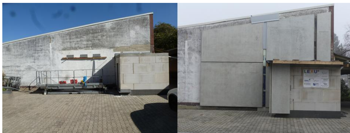
Figure 47: Implementation of the demonstration façade at KOMZET BAU in Bühl – initial condition (left) and with mounted sandwich façade elements (right). Source: Uwe Schneider, KOMZET BAU Bühl
