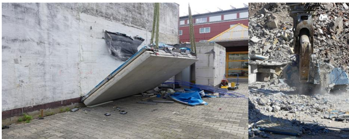
Figure 48: Dismantling (left) and recycling (right) of the sandwich façade elements. Source: Uwe Schneider, KOMZET BAU Bühl
