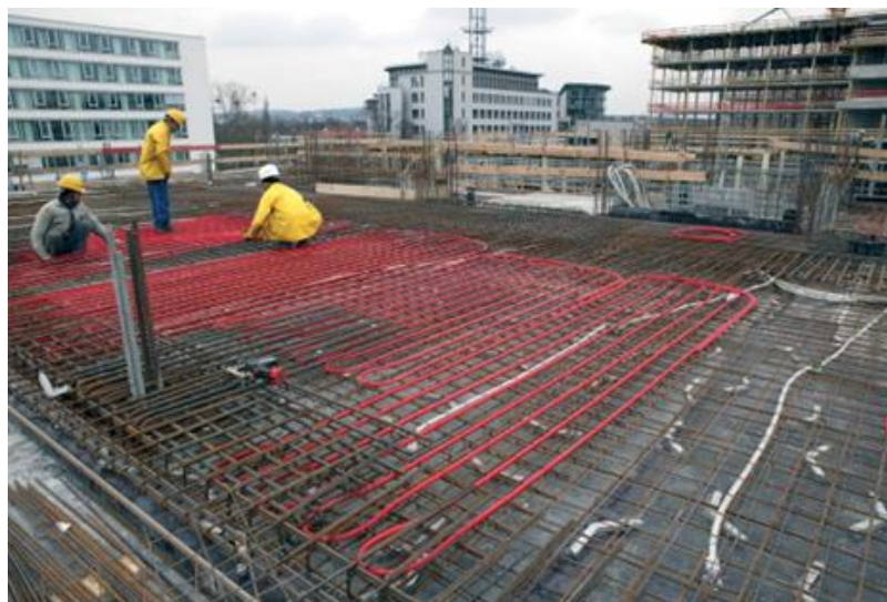
Figure 5: During component activation, a system of water-conduction pipelines is laid into concrete components via manual labour on site. Source: Innogration GmbH
