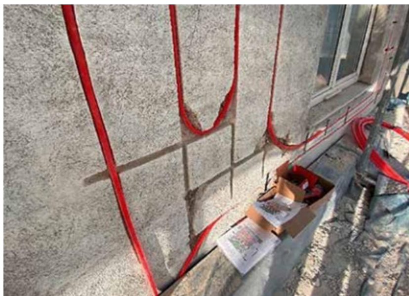
Figure 29: Heating pipes in the exterior wall, before the thermal insulation is installed. Source: IBR&I – Institute of Building Research & Innovation
