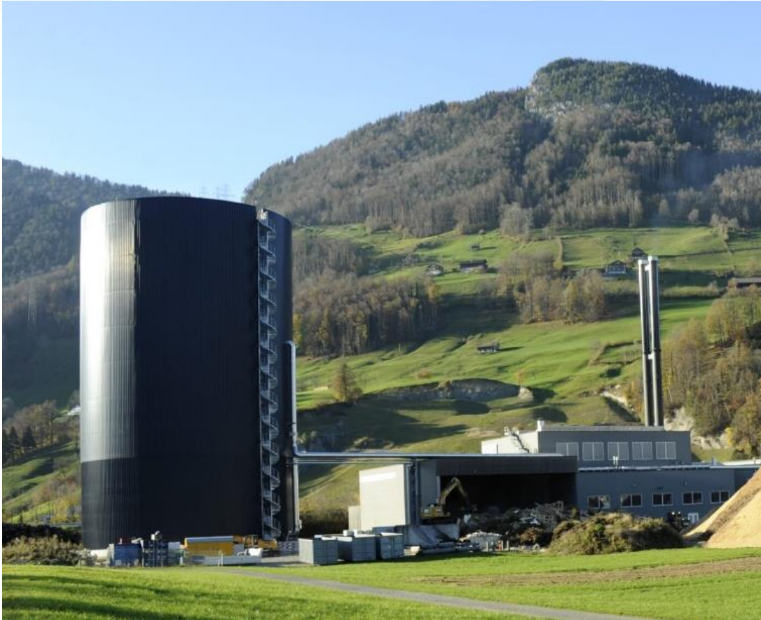
© AgroEnergie Schwyz AG. 28'000 m 3 unpressurized water tank.
