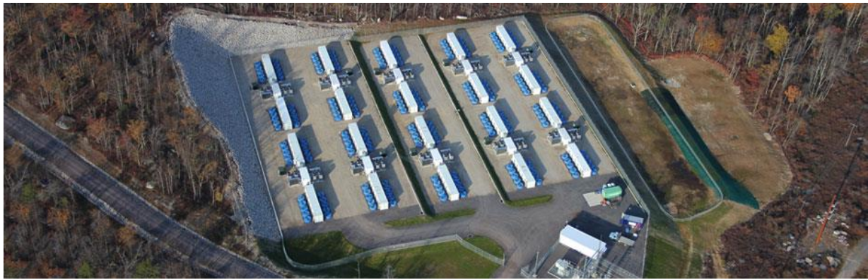
Figure 4: 20 MW storage for frequency regulation in Pennsylvania, USA (© Beacon Power)
