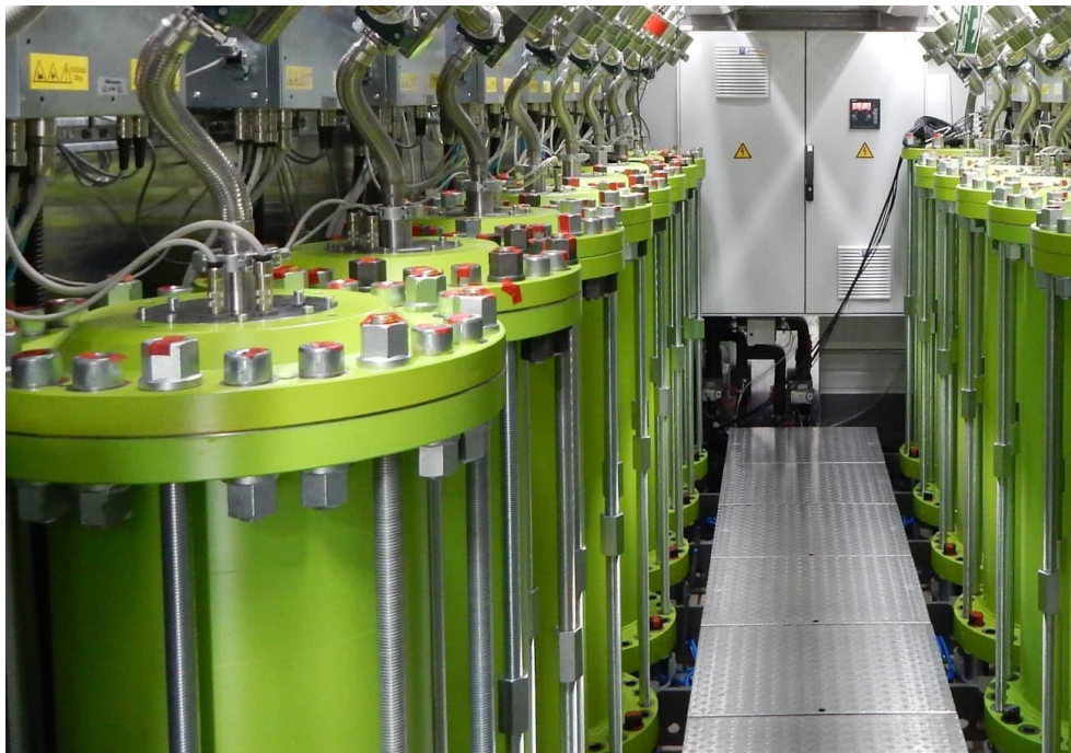
Figure 1: Inside of a FESS module (© STORNETIC)
