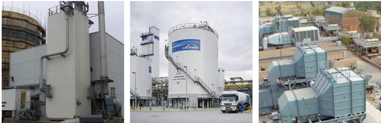
Figure 2: Condenser, cryogenic liquid tank for 350 MWh el , hot gas expander (l.t.r.) (© Linde)
