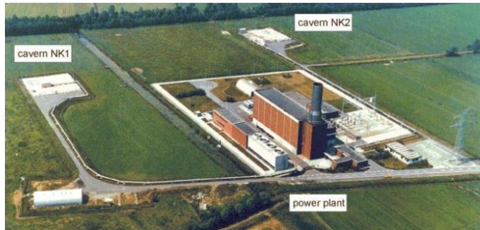
Figure 3: CAES plant in Huntorf, Germany (© E.ON Kraftwerke GmbH)
