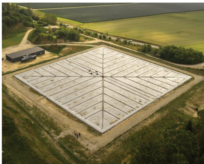
Figure 4: Pit heat storage in Dronninglund, Denmark (© PlanEnergi)
