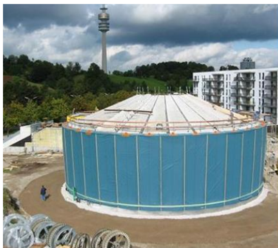
Figure 3: 6,000 m 3 seasonal heat storage tank in Munich during construction and after being completely buried in a hill (© ZAE Bayern)
