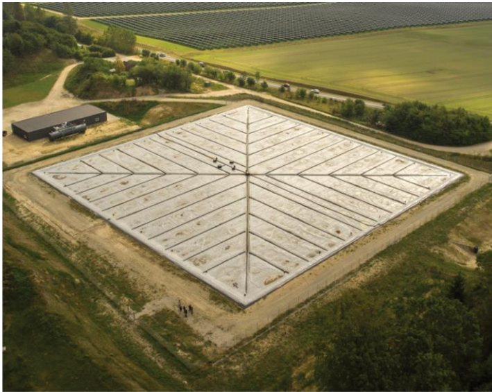
Figure 4: Pit heat storage in Dronninglund, Denmark (© PlanEnergi)
