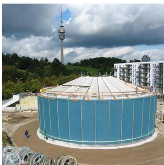
Figure 3: Seasonal local heat storage (6,000 m 3 ) developed by ZAE Bayern, charged using solar heat at 48 % coverage (3,000 m 2 of collectors)
