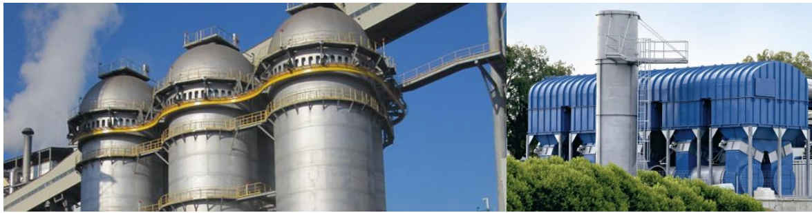
Figure 1: Cowper in a blast furnace process (l.), thermal-oxidative exhaust air purification (r.) (sources: [1], [2])
