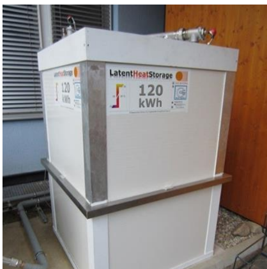
Figure 4: Latent heat storage for recooling of an absorption chiller used in solar air conditioning (left, source: ZAE Bayern), PCM crystallising on heat exchanger during discharge of storage (right, source: ZAE Bayern)
