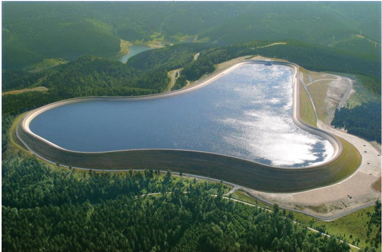
Figure 1: Upper reservoir of Goldisthal Pumped Storage Plant in Germany (© Vattenfall)
