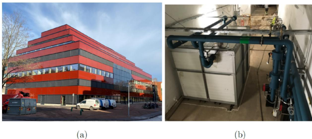
Figure 5-5: "A working lab" (AWL) office building (a) and PCM TES installation located in the basement of AWL (b) [68].
