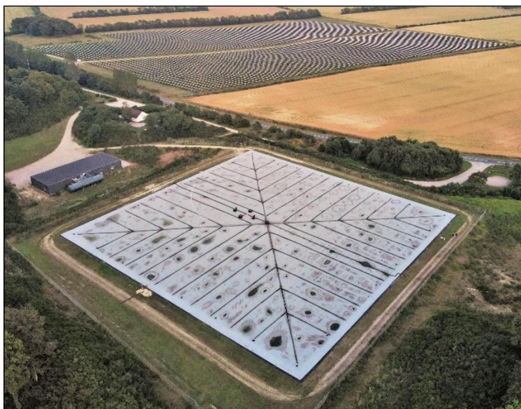
Figure 7-5: Aerial view of the PTES and solar collector field in Dronninglund, Denmark [75].
