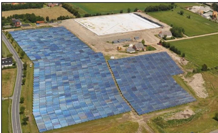
Figure 7-7: Aerial view of the PTES and solar collector field in Marstal, Denmark [77].
