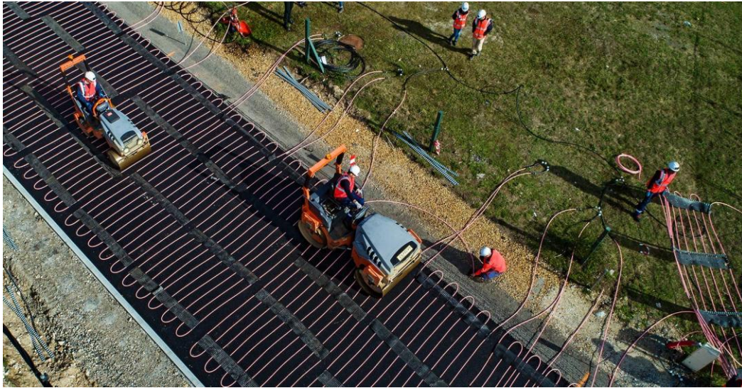
Figure 10. Pipe placement in Power Road project (Power Road website)
