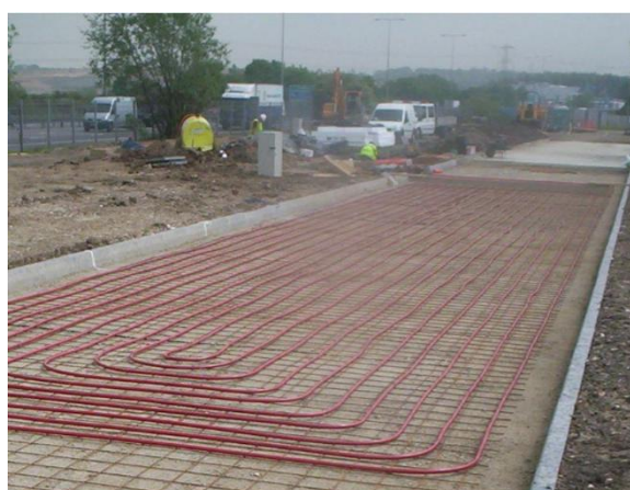
Figure 9. The construction stage of HHP without grid support (left) Power Road where the tubes are placed in grooves in the previously installed layer ( Vinci 2019 ), (right) ICAX TRL project where the pipe network is connected to a steel square mesh using metal pins ( ICAX )
