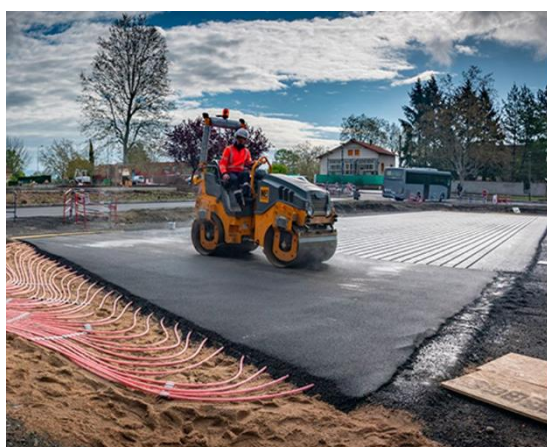
Figure 9. The construction stage of HHP without grid support (left) Power Road where the tubes are placed in grooves in the previously installed layer ( Vinci 2019 ), (right) ICAX TRL project where the pipe network is connected to a steel square mesh using metal pins ( ICAX )
