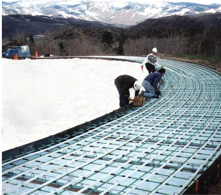
Figure 24. Pipe installation in concrete with spacer holders (Uponor project) ( Uponor 2015 )
