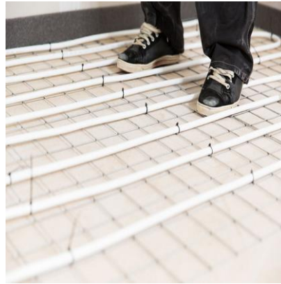
Figure 7 pipes are tied with the wire mesh
