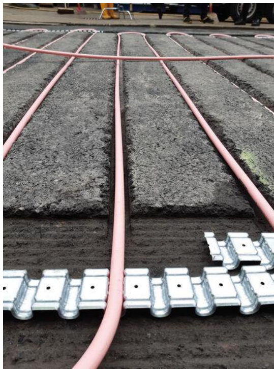
Figure 11. Pipe placement using metal spacers (from Eurovia Germany website)
