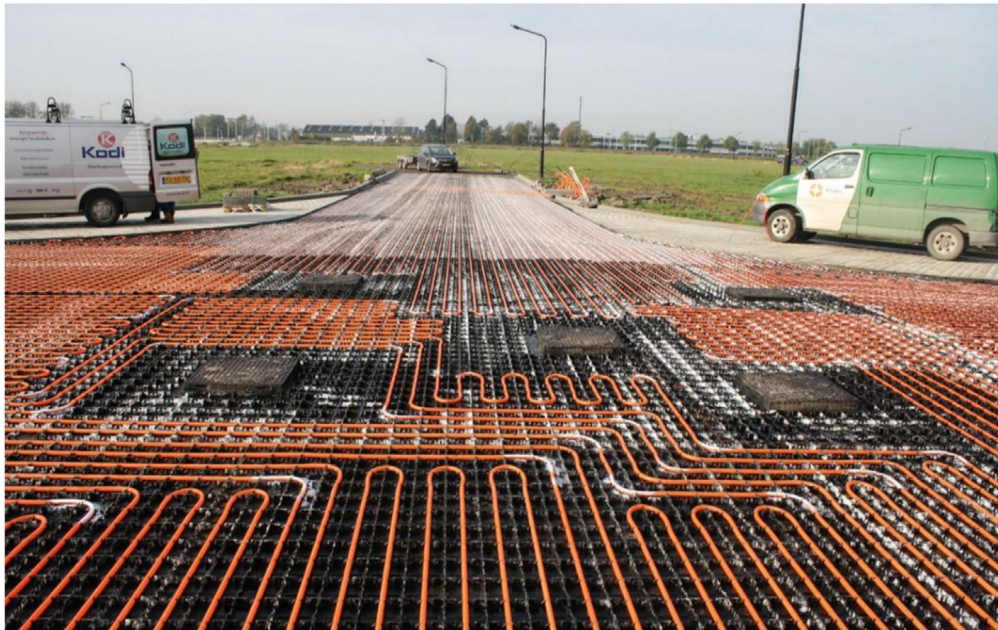
Figure 4. The construction stage of HHPS with grid support (Ghalandari et al 2021).
