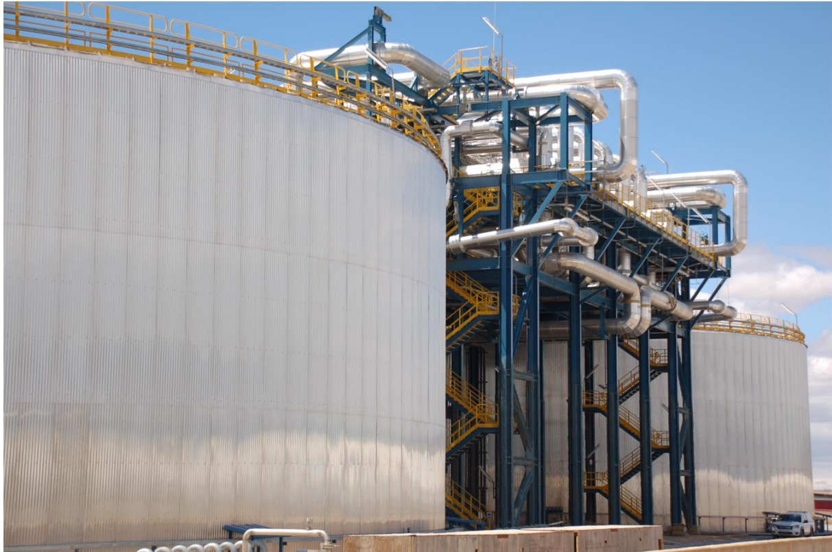
Figure 2: Liquid salt storage in a CSP plant (source: Andasol 3)
