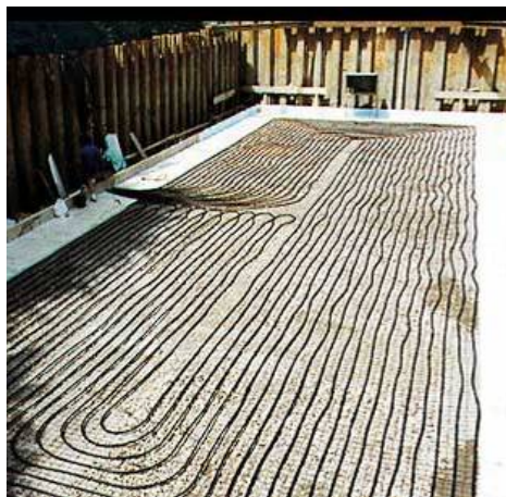
Figure 4. Completion of the foundation absorber
