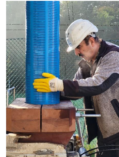
Installation PVC filter screen (in observation well P1)
