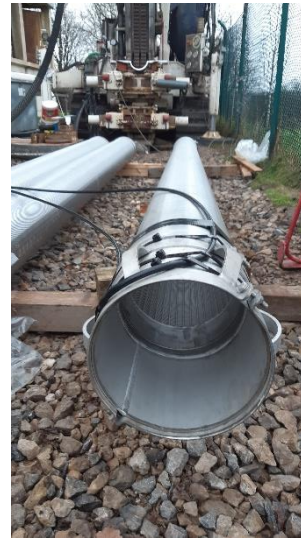
Wire wrapped screen tubes for MTES well P2
