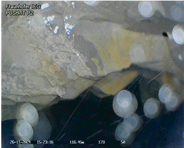
Tapping into flooded mine void (via camera inspection)
