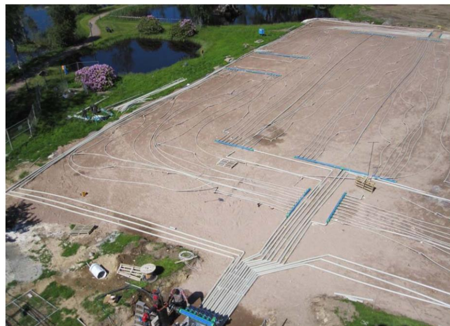
Picture showing the piping and manifolds of some sections of the BTES in Emmaboda during installation in 2010
