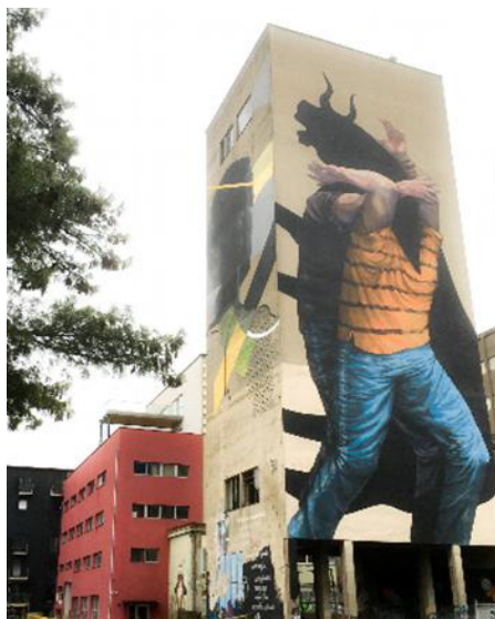
Picture of Demo building
