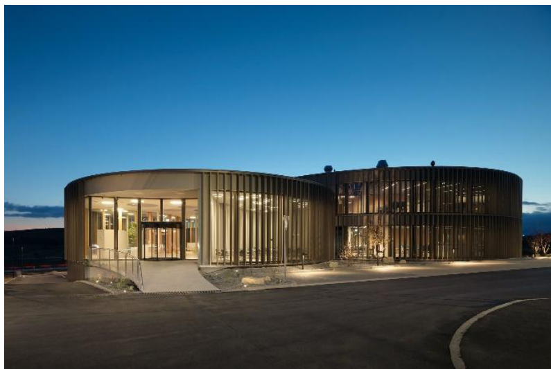
Picture of Demo building
