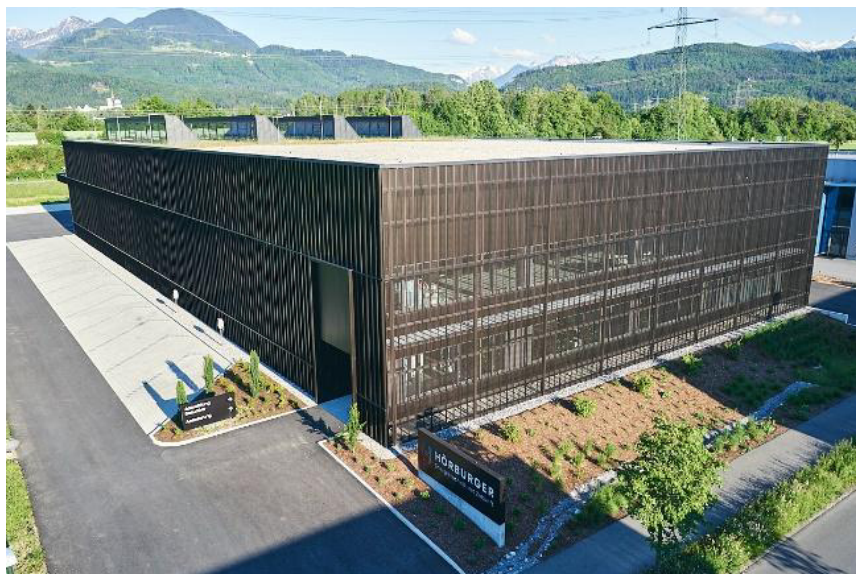
Picture of Demo building
