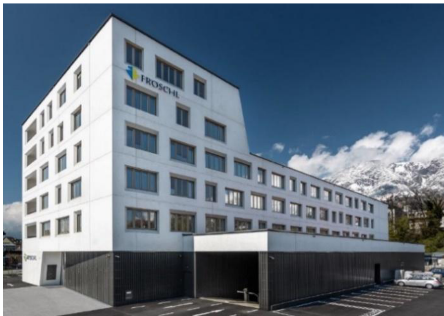
Picture of Demo building
