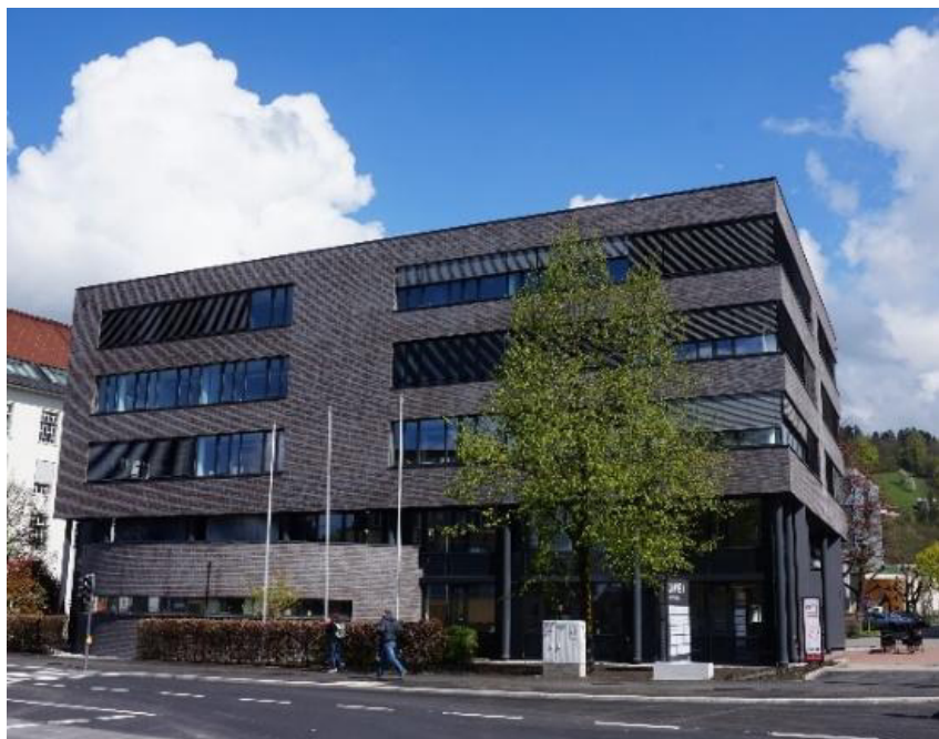
Picture of Demo building
