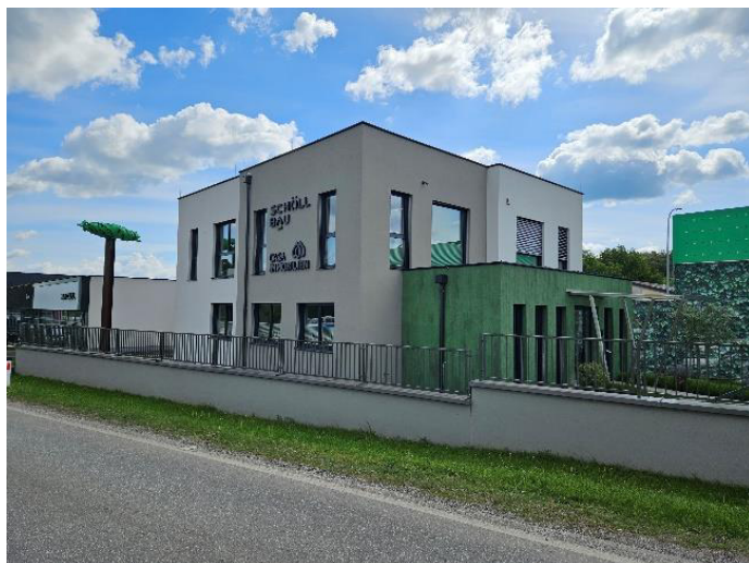
Picture of Demo building
