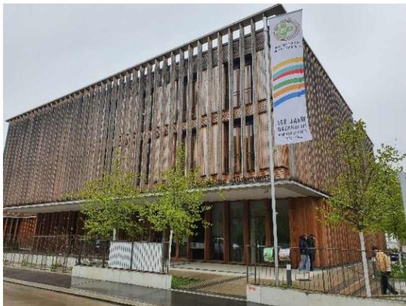
Picture of Demo building
