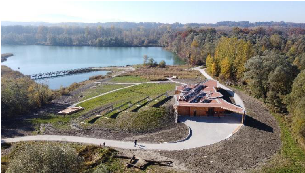
Picture of Demo building
