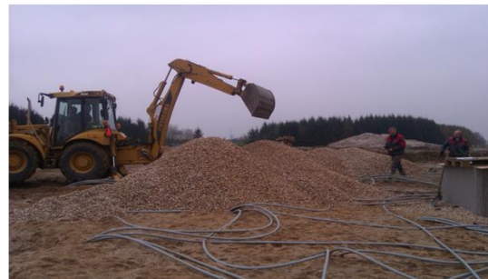
BTES in Brædstrup, main implementation steps. Pictures: PlanEnergi
