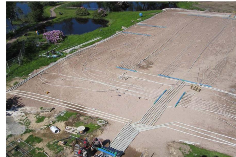
Picture showing the piping and manifolds of some sections of the BTES in Emmaboda during installation in 2010
