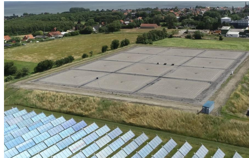
PTES from Marstal district heating (photo: Aalborg CSP)
