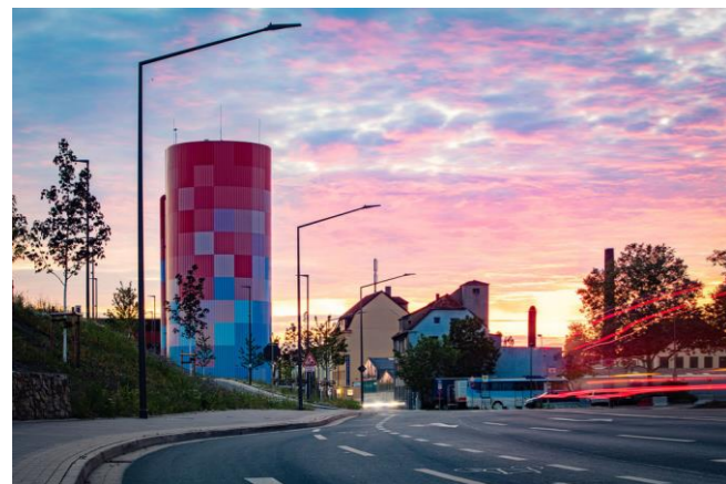
TTES from Stadtwerke Detmold 1'850 m 3 of water
