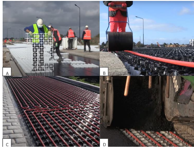
Fig. 4. Using plastic mesh for positioning the pipe. (www.ooms.nl)
